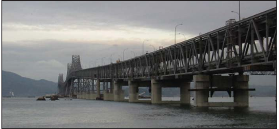
The Richmond-San Rafael Bridge
