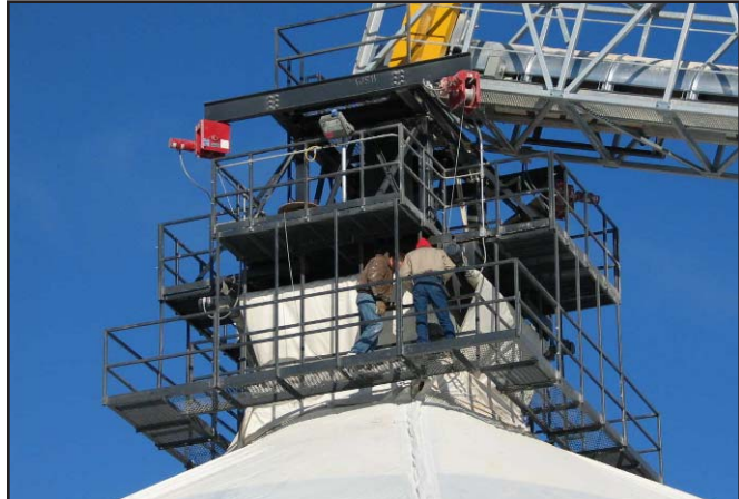
Thern winches mounted on the perimeter of a tower.
